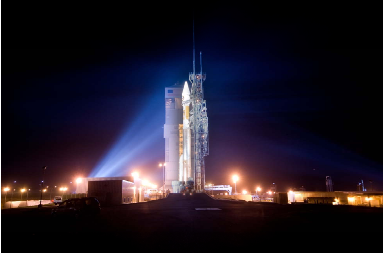
Figure 7.2.3-2: Space Launch Complex 3-East
